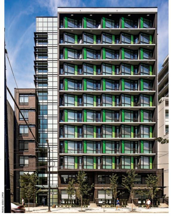
Each apartment facing Howe Street was positioned at a slight angle. The resulting saw-tooth appearance provides visual flair (by breaking up the monotonous nature of apartments stacked on top of each other), enhances privacy and reduces solar glare.
